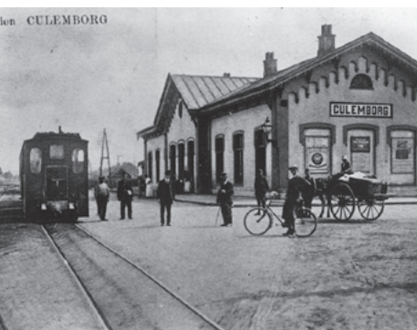
Eindpunt Culemborg Station
