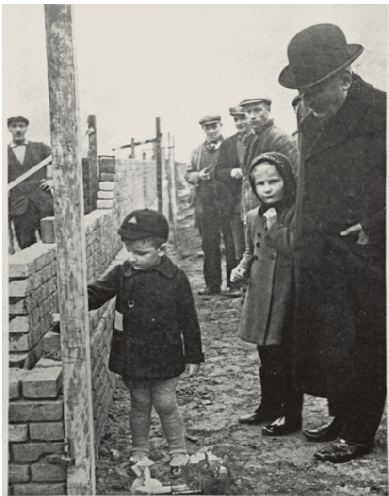
Laying of the foundation of the C.V. Knitwearfactory Pehavee at Veenendaal by Bert Heij on the 13th of February 1939 in the presence of his grandfather the late Mr. Lammert Heij
